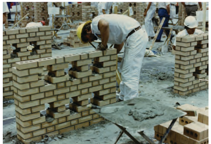
Students practice bricklaying in masonry class.
