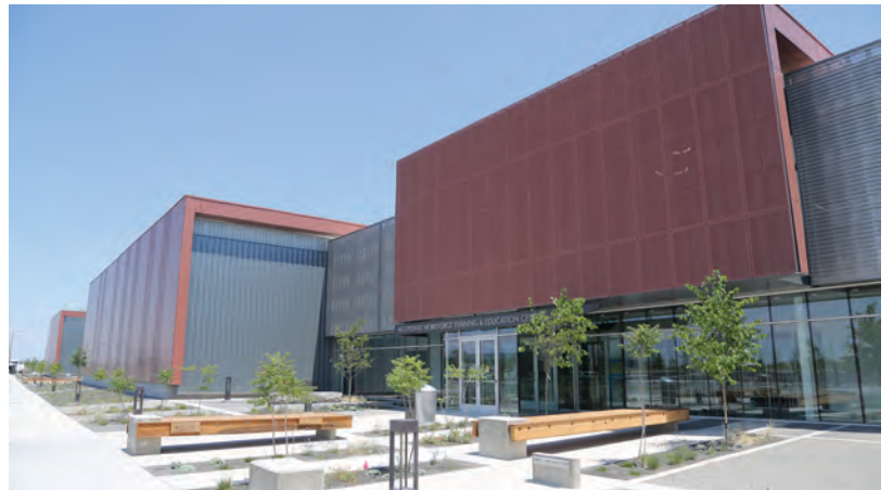
The Westpointe Workforce Training & Education Center opened in fall 2018.
