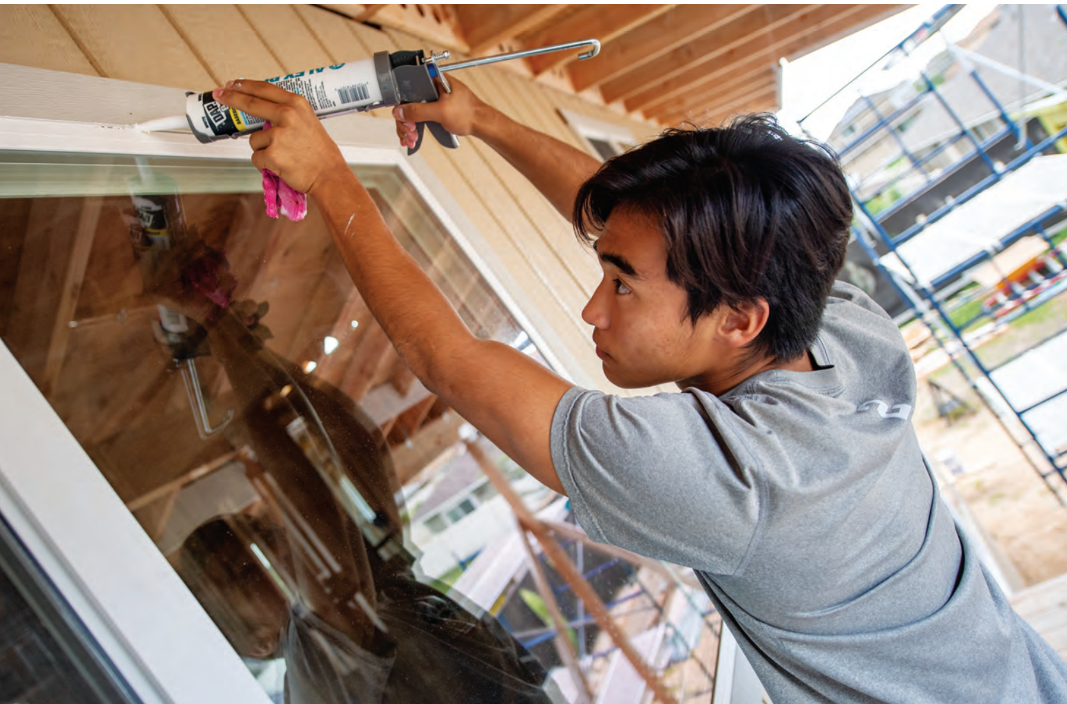
James Fujita '21 adds caulk to a window.
